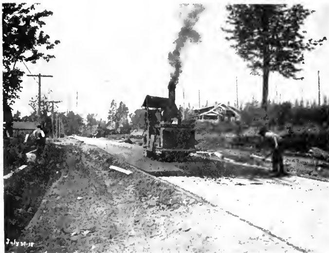
Ten ton roller on surface work, Marine Highway, B. C.
